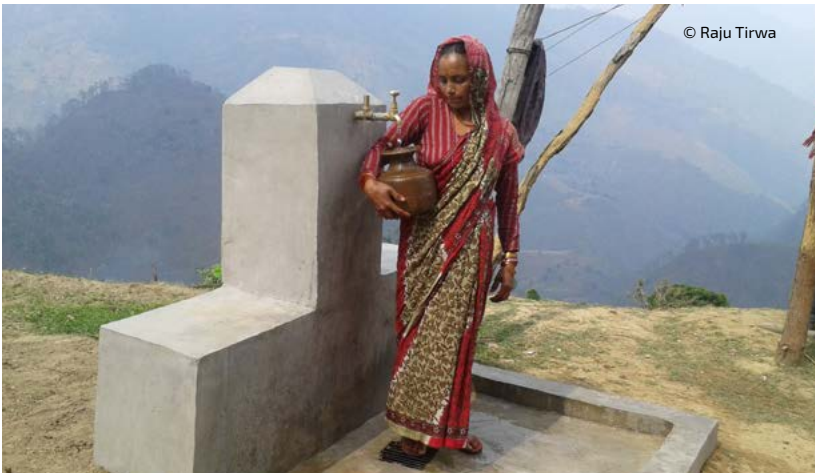
Water access point in the Dadeldhura district in Nepal, created during Phase II of the RVWRMP project supported by the European Union.
